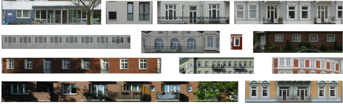
Figure 3: Examples of the variety of floors with the domain. Because the floor where automatically extracted using the annotations also floor that are only partially visible, such as the floor with only one window visible are in the training and testing data.
