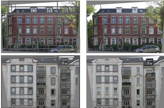
Fig. 8. Complete annotated images alongside automatically detected structures of the classes Entrance , Balcony and Window-Array
